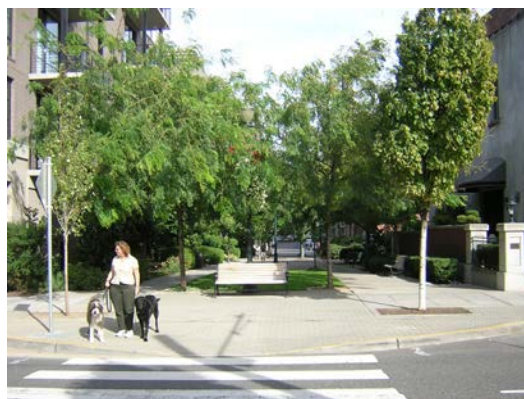
BULBOUTS WHERE UNIVERSAL STREETS MEET VEHICULAR STREETS FACILITATE PEDESTRIAN CROSSINGS AND INCREASE VISIBILITY
