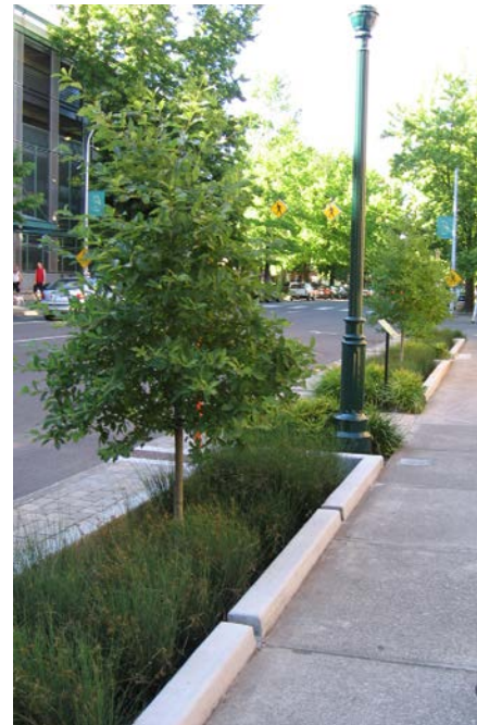
CONSTRUCTED STORMWATER PLANTERS MANAGE RUN-OFF WHILE PROVIDING A VISUAL AMENITY WITHIN THE STREETSCAPE
