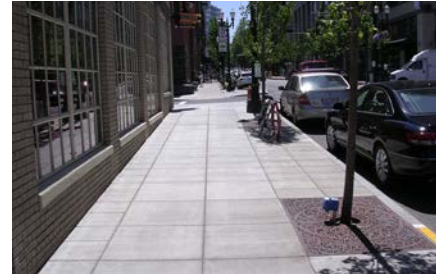
CONCRETE IS THE STANDARD SIDEWALK TREATMENT THROUGHOUT THE DISTRICT. A LARGER PATTERN IN THE CLEAR ZONE BORDERED BY A SMALLER PATTERN IN THE BUILDING FRONTAGE AND FURNISHING ZONES HELPS TO GIVE DEFINITION AND CREATE VISUAL INTEREST
