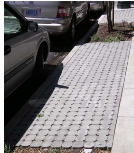
ALONG RIVERFRONT AND GRAND, SPECIAL PERMEABLE PAVERS SHALL BE USED WITHIN THE FURNISHING ZONE TO HELP VISUALLY DISTINGUISH THESE TWO IMPORTANT STREETS. THESE PERMEABLE PAVERS WILL ALSO HELP TO MINIMIZE STORMWATER RUNOFF
