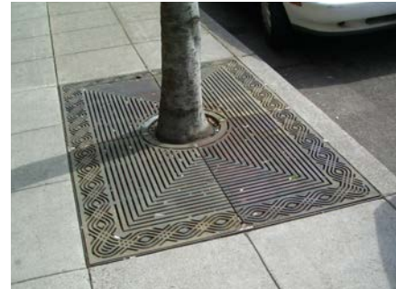
EXAMPLE OF CAST IRON STREET TREE WELLS.
